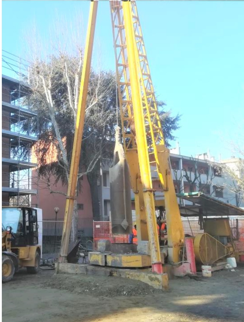
Geothermal wells drilling
