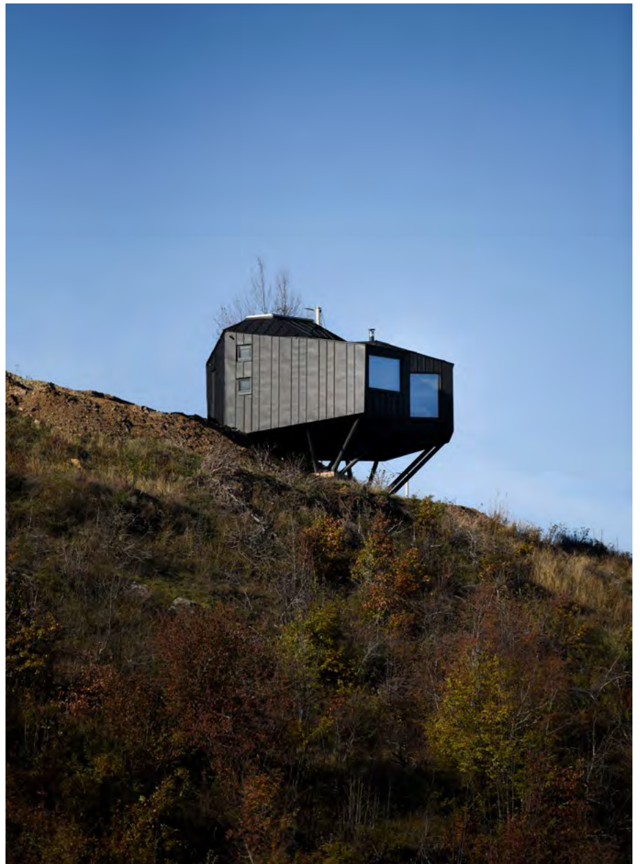
HUT SPACE, Novo Brdo, Kosovo Architect: Visar Geci Photo: Visar Geci
