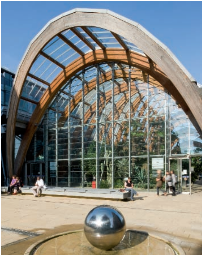
Sheffield Winter Gardens and Gold Route © CABE/David Millington Photography Ltd
