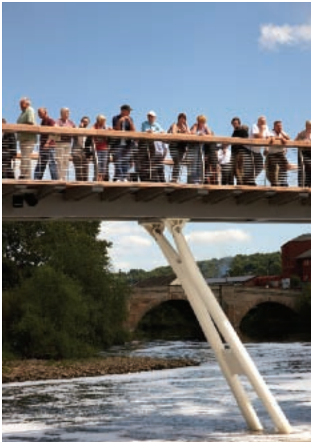
Castleford footbridge © Tim Soar
